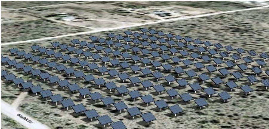
20+MW Utility Plants
